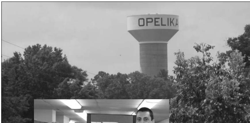
OPELIKA WATER TOWER
